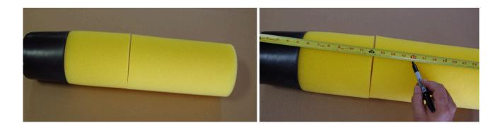
3. Using a bread knife or hacksaw with fine-tooth blade, carefully cut the additional foam section to the desired length.
