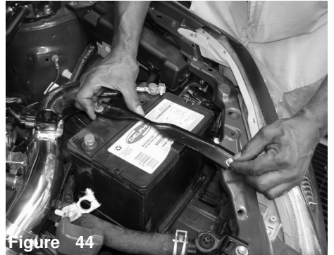
Figure 44 The battery tie down is now placed over the battery to hold it in place.
