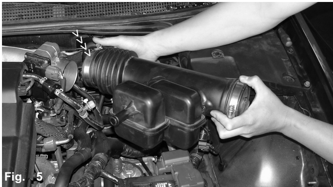
Fig. 5 Loosen clamp at the throttle body and remove the air intake duct. At this point, it will be necessary to remove the front bumper. Remove 9 clips on top of the bumper, two 10mm screws on each side of the bumper, four additional sheet screws and 5 plastic clips.
