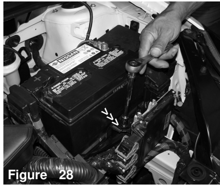
Figure 28 The m8 bolt on the metal battery tray is now fastened.
