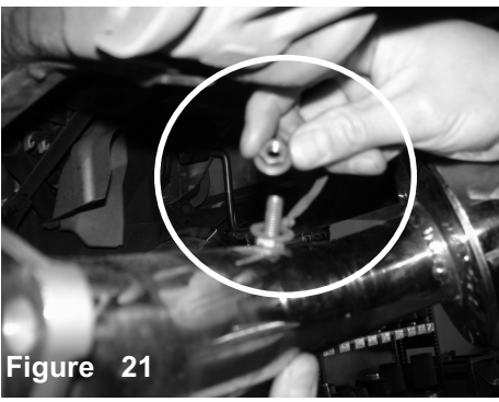
Figure 21 Place a supplied M8 nut to the welded bolt and secure the grounding wire to the Injen exhaust system.
